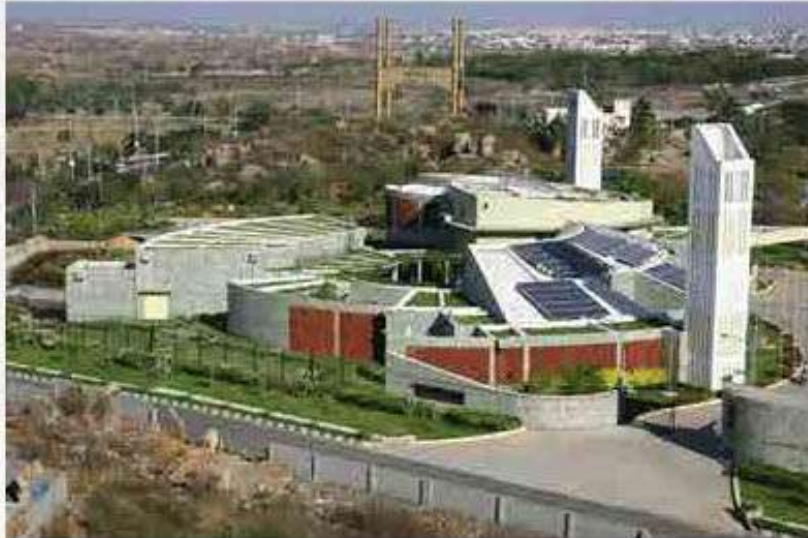
The first LEED platinum-rated building in India - CII-Sohrabji Godrej Green Business Centre
